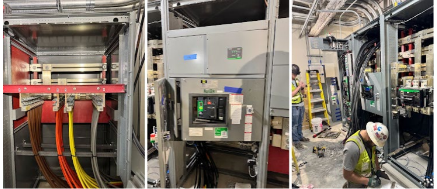
Primary electrical room work in prep for PUD service
