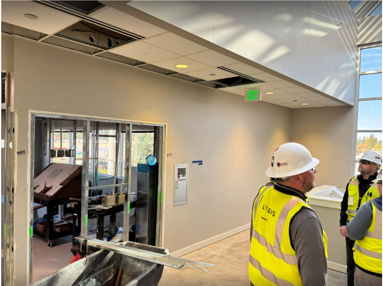
A3 Wall at top of Stairs. This will be a solid wall used as a backdrop for employee photos, as this idea originated from one of our employees. (Fire Extinguisher will be relocated)
