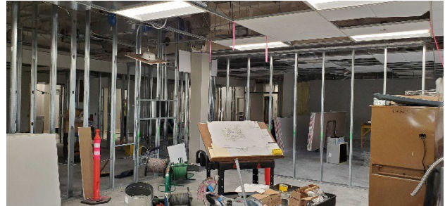
Building A - Floor 2 West
