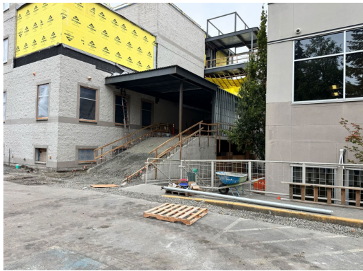
Employee Entrance awning installed
