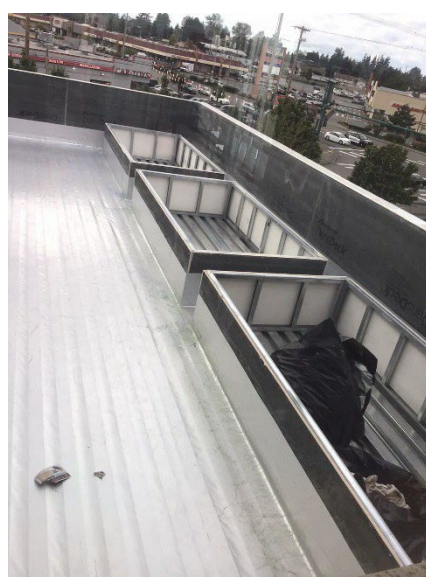
New Roof above Dispatch with Skylights
