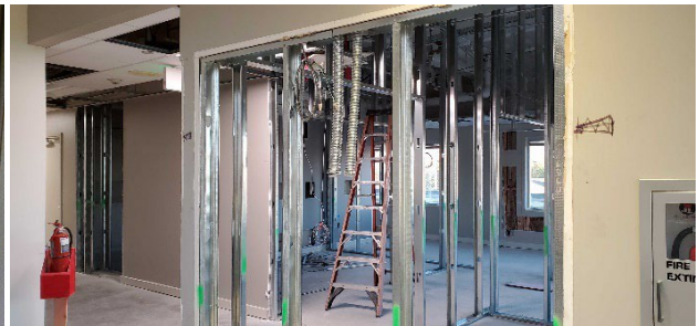
Building A - Floor 4 West
