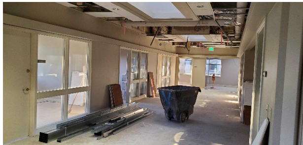
Building A - Floor 3 East – Reusing existing offices
