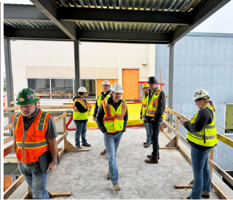
Top Floor Building Connector partially complete
