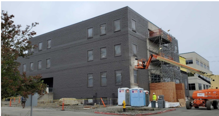
Building B – Exterior Painting view facing north.
