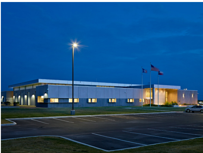
Building Entry - Night view
