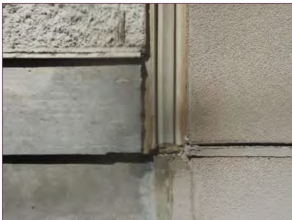
Photo 5.1.1.1-5: Base of seismic joint, sealed, typ
