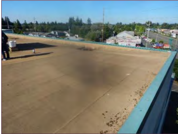
Photo 5.1.1.2-1: Typical roof membrane, minor
