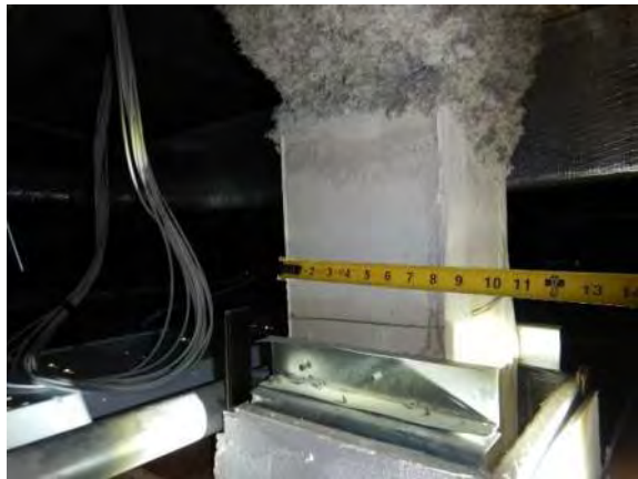
Photo 5.2.1.2-3: 8-inch-wide column (including drywall framing) at grid 2-D
