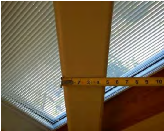
Photo 5.2.2.3-1: 5x5 HSS at 4th floor braced frame
