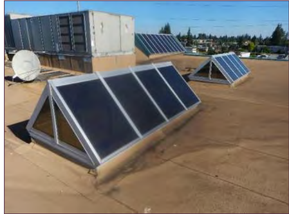
Photo 5.1.1.3-2: Small skylights, east side
