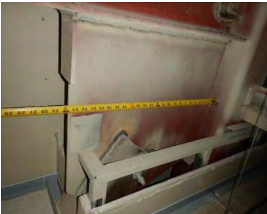
Photo 5.2.2.3-3: Diagonal brace to column connection
