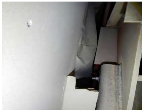
Photo 5.2.2.3-4: Stiffener plate at back side of gusset plate
