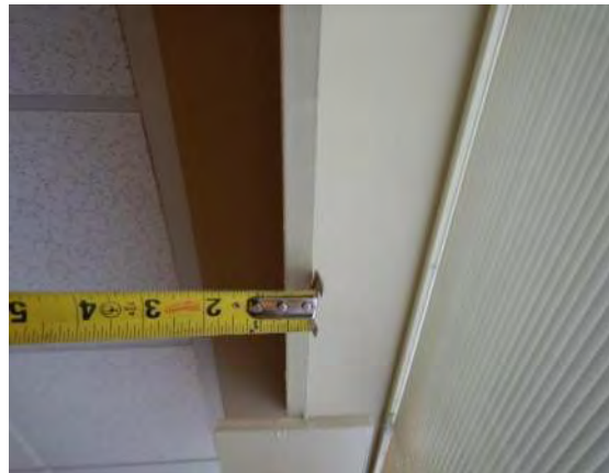
Photo 5.2.2.3-2: ½ inch gusset plate at 4th floor braced frame
