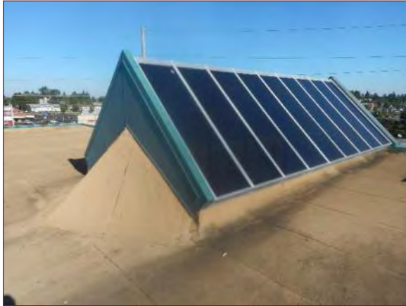
Photo 5.1.1.3-1: Primary skylight, north side
