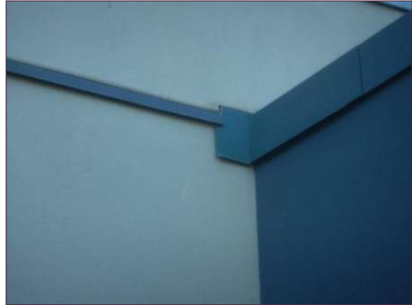
Photo 5.1.1.1-4: Coping metal saddle integration
