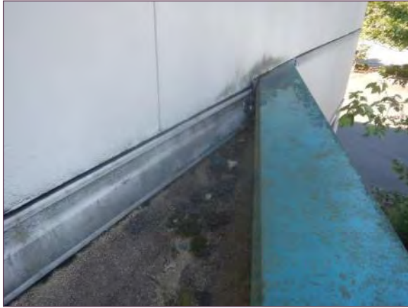
Photo 5.1.1.4-3: Roof transition at west side canopy
