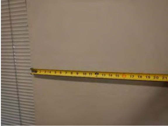
Photo 5.2.1.2-1: 16-inch stud spacing at shear wall SW4
